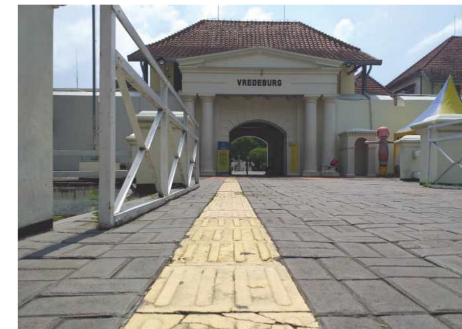
Foto Fasilitas Guiding Block di Museum Benteng Vredenburg Yogyakarta (Foto: Dyota Hayu Mahardhika)
